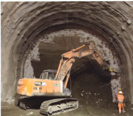
Excavation of section C1.
