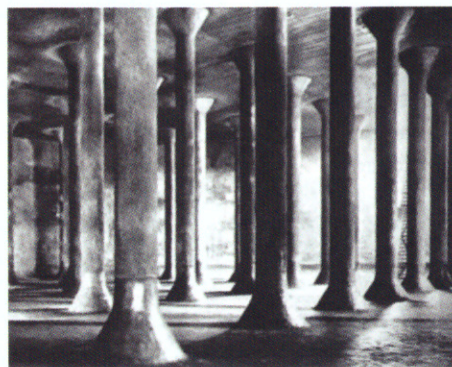
Internal view of the tank (Argiroffi, 2008).
