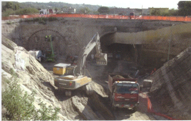
Northern Portal site where jet-grouting was used to support excavation slopes.
