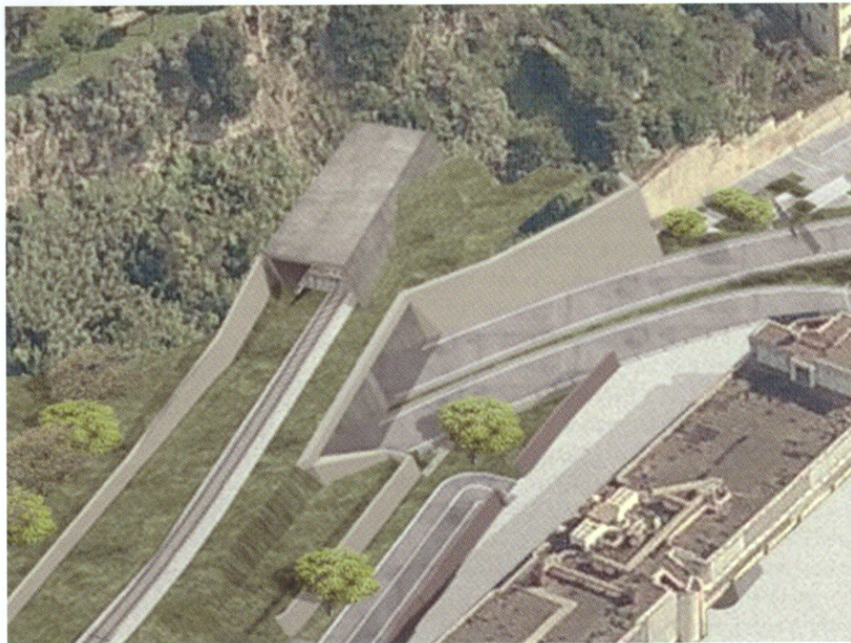
Southern tunnel portal towards the port.
